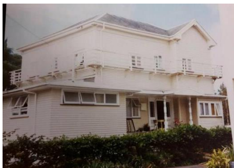
Boarding House, Corbett Scott Ave, Epsom
