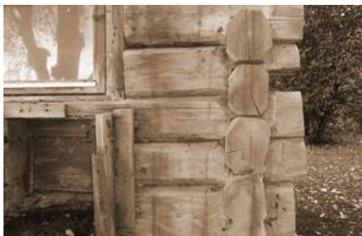
All cabins, houses and farm buildings were made with interlocking logs like this.
